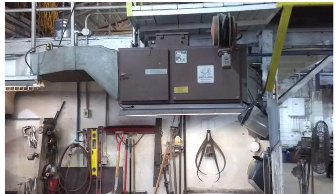
Source capture system to serve grinding table
