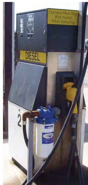
VF-61 connected to a diesel fuel dispenser
