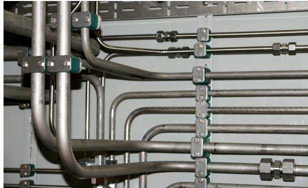
and incorporating elbow fittings—providing “give” to the line. With this fix, the system no longer leaked.
