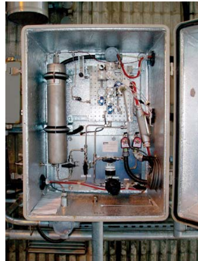
Sarnia's SHS layout features two separators and valves that direct sample and reference gasses.
