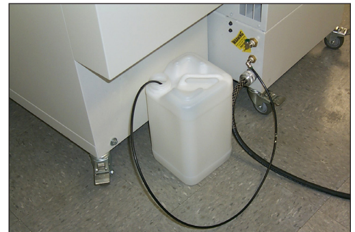
Figure 12 Compressor Drain to Disposal Container
