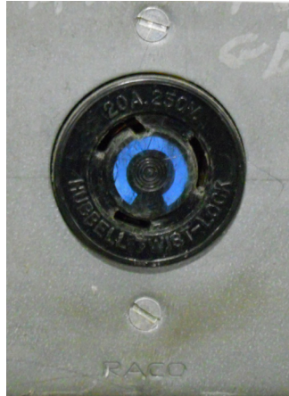
Figure 9 Compressor 20 Amp, 250 V Receptacle for NA model
