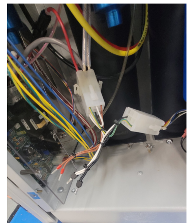
Figure 6 - Controller Harness Installation
