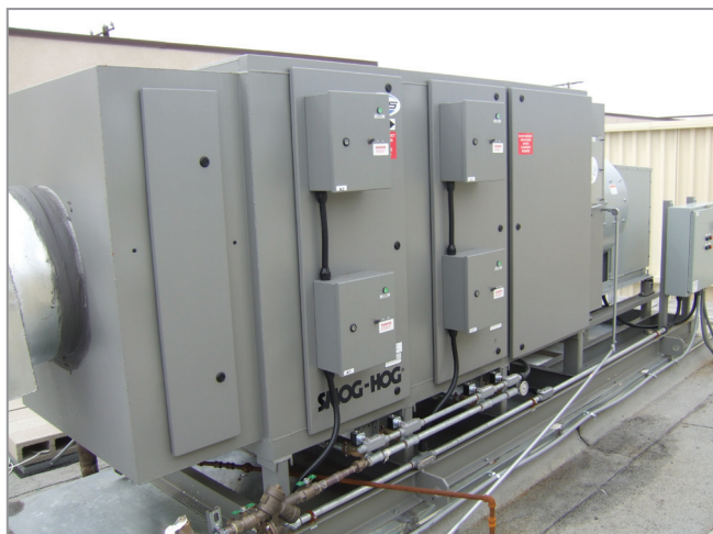
For heavy particulate loading such as wood-fired cooking or smoking applications, multiple passes can be used to achieve higher levels of removal efficiency.
