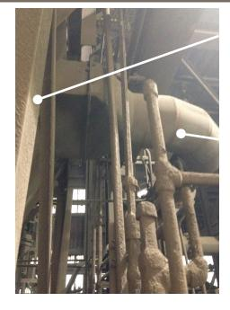
Ductwork inlet design forces air to left side of the baghouse
