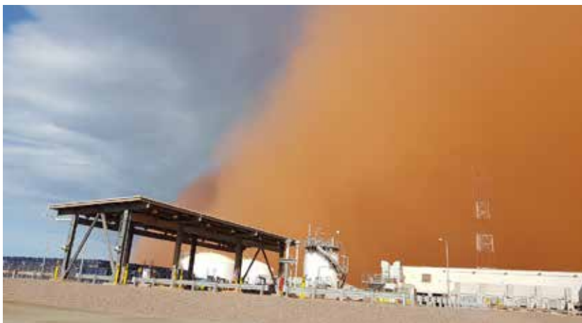
Fig. 3. Photo of sandstorm taken at an LNG facility in Western Australia. If there are high levels of dust, like those often found in desert regions, care also needs to be taken that the coalescers do not get blocked, which may cause pressure spikes or force the coalescer out of place, rendering its protection useless.
