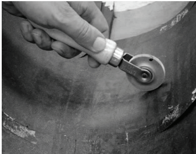
Figure 3. Rubber Stitching after Application
