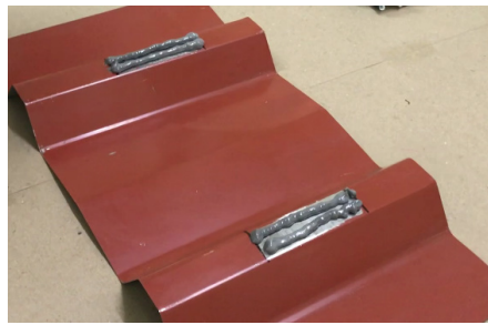
Figure 5. Apply adhesive to grinded area
