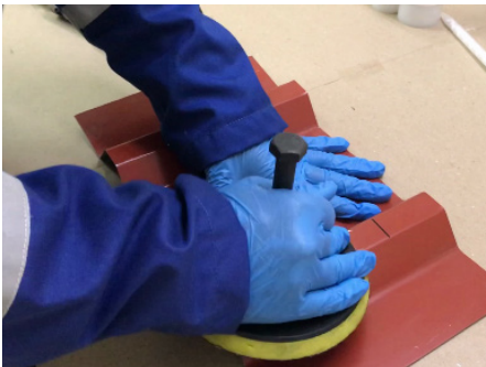
Figure 2. Grind application area only
