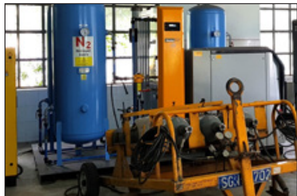
Parker NITROSource PSA with 300barg nitrogen booster system for portable nitrogen cart cylinder filling, within airline maintenance bay
