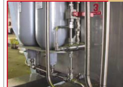
... and at the hydraulic accumulator which is used to store energy for peak demands.
