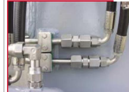
Safety and environmental protection are at the fore in the design of davits. VESTDAVIT equips the entire hydraulic tubing system with O-Lok® fittings. Some examples are adjustable O-Lok® fittings at the cylinder...
