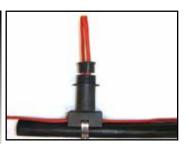
Insert heating cable through tubing bundle standoff and grommet as shown. 8 inches of cable should extend past the grommet. If only two cables are entering the kit close off the remaining grommet opening with the appropriate grommet insert. Attach the standoff to the bundle with a SS hose clamp as shown.
