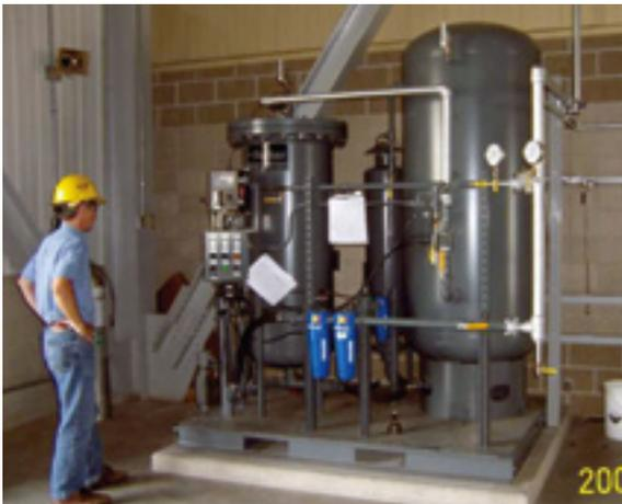
**25. Nitrogen generator skid** saves cost of rented, vendor-supplied compressed  $\text{N}_2$  bottles
