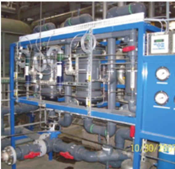
**27. Gas-transfer membrane skid** deoxygenates makeup water before it enters the steam cycle
