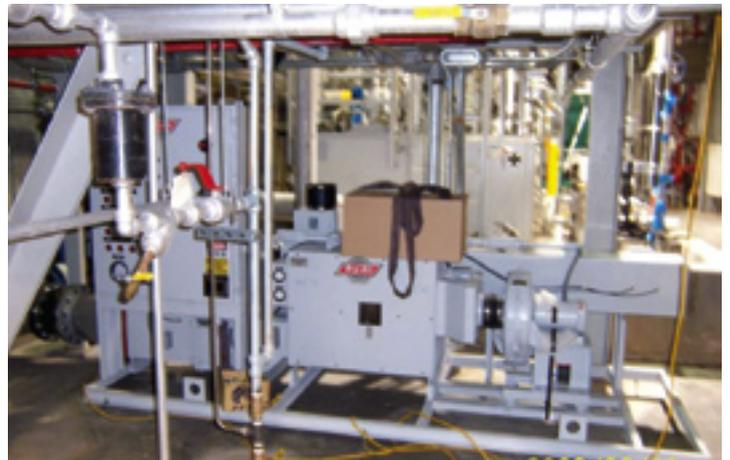
**26. Desiccant wheel dehumidifier** prevents pitting of LP steam-turbine blades which could lead to CF or SCC
