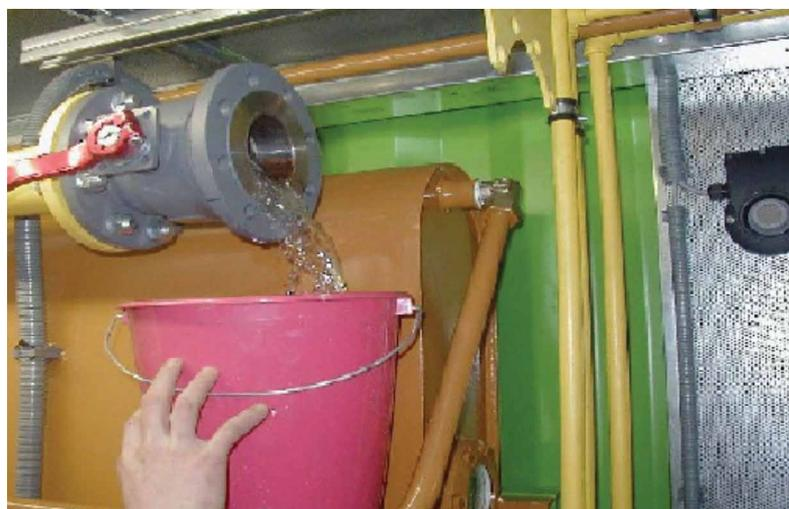
Fig 1 – Water condensate in biogas pipework
