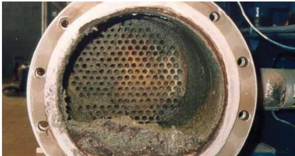
Fig 3 – Pipescale in heat exchanger
