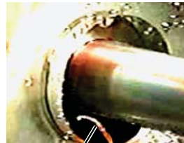
Water Being Pumped into the Bearing Cavity
